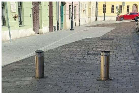
Figure 6. Smart pillar preventing entry
